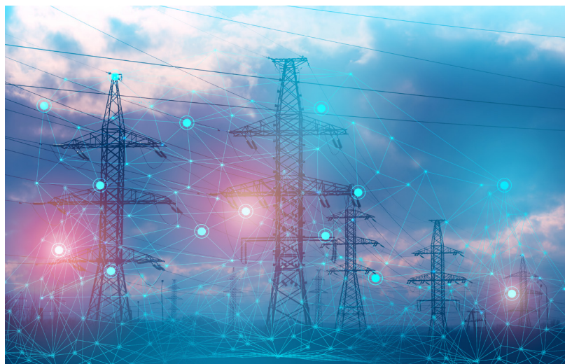
Artificial intelligence is being used to increase reliability and reduce losses and accidents during the transmission of electrical energy. © AdobeStock
